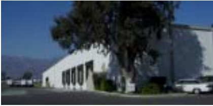
Clement Pappas California facility
